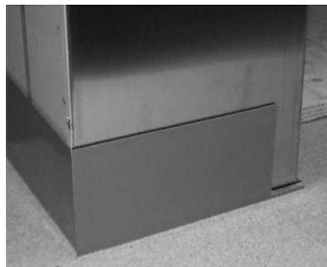
This detail shows the notch in the U channel with the corner panel in place. Therefor allowing the gasket to seal against the panel.
