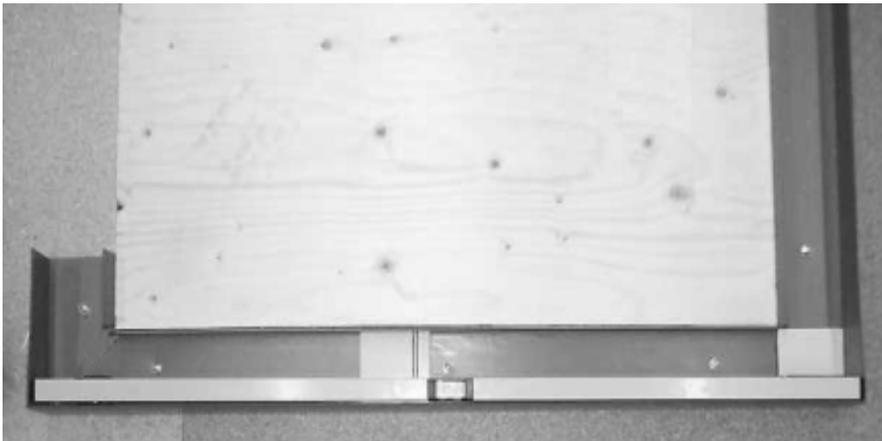
It is recommended that there should be no more than 3mm tolerance in the floor level as this can effect the correct location of the locking panels.
