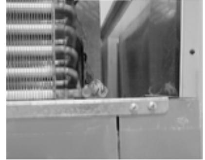
With the ceiling panel secured in place seal the internal joints with silicone sealer. Insert the buttons into the lock holes.
