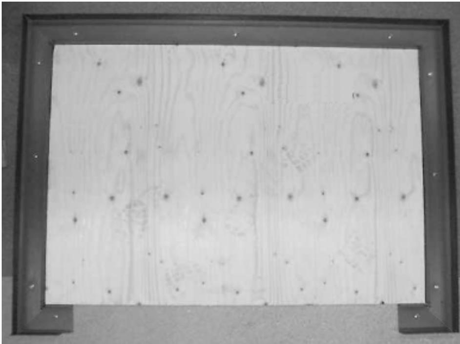
Once you are satisfied with the level the U channel can be rawl-plugged or hilti-nailed into position ensuring it is sealed with silicone sealer between the floor and the channel to prevent moisture penetration.
