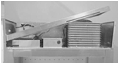
With the ceiling panel in place slide the galvanised angle bracket into place (see fig 4). Secure in place using the screws provided (see fig 5 and 6).
